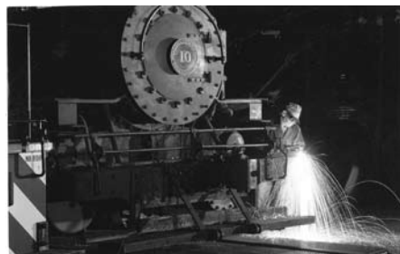
Conn. Eastern RR Museum member Bob Hassett does some night repairs on Steam #10.
